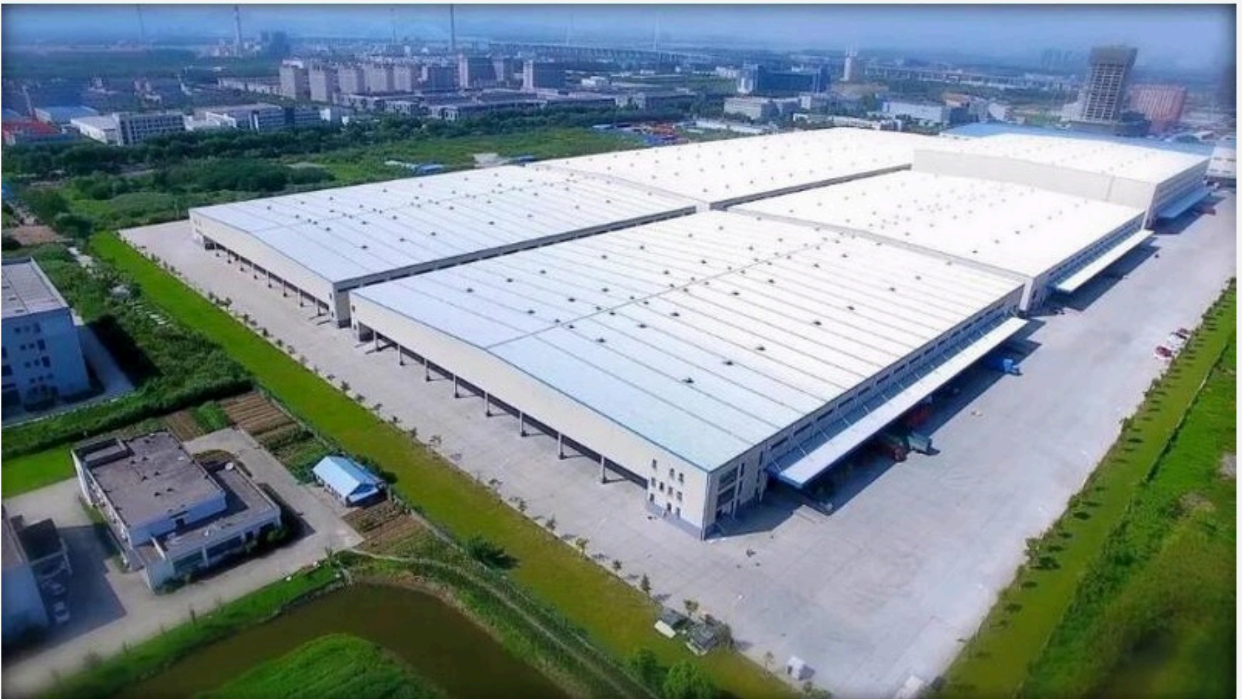
Distribution Centre: PUF Roof Panel
