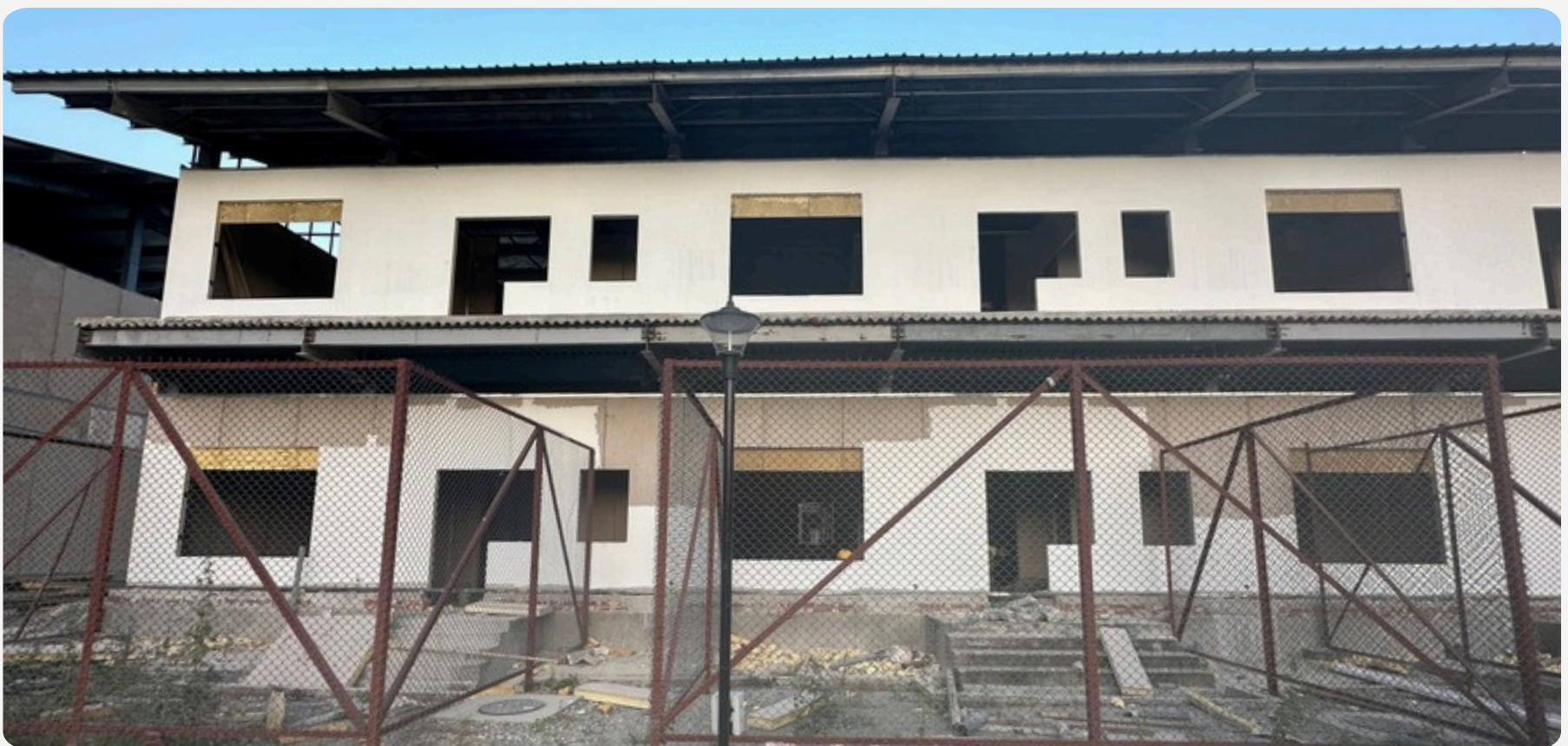
Windows Cutout using HandSaw, and applied putty/primer
